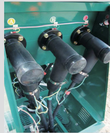
Fuzhou Railway Separable Connector Installation SiteG
