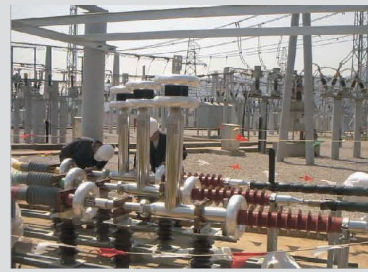
Yunnan Cable Termination Installation Site
